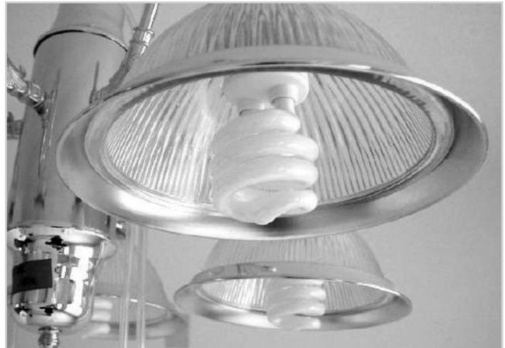
Figure 1 Compact fluorescent lamp in a test house
