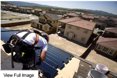
Construction workers from SunPower Corporation install integrated SunTiles onto the roofs of new homes under construction in San Ramon, California.
